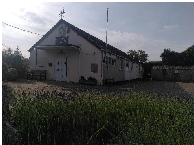
Recreation Hall, Long Hanborough
